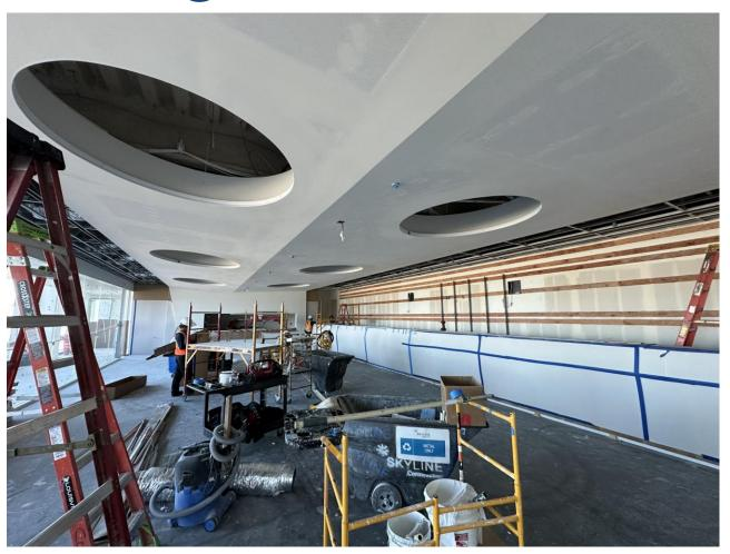
Level 5's Public Hearing Room has evolved. The raised dais is now fully protected, with acoustical ceilings installed and drywall finish underway.
