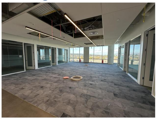
Flooring, ceiling, storefront, and doors are all installed and final cleaning is underway.
