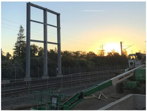
Installation of steel gantry for traction power station in Palo Alto
